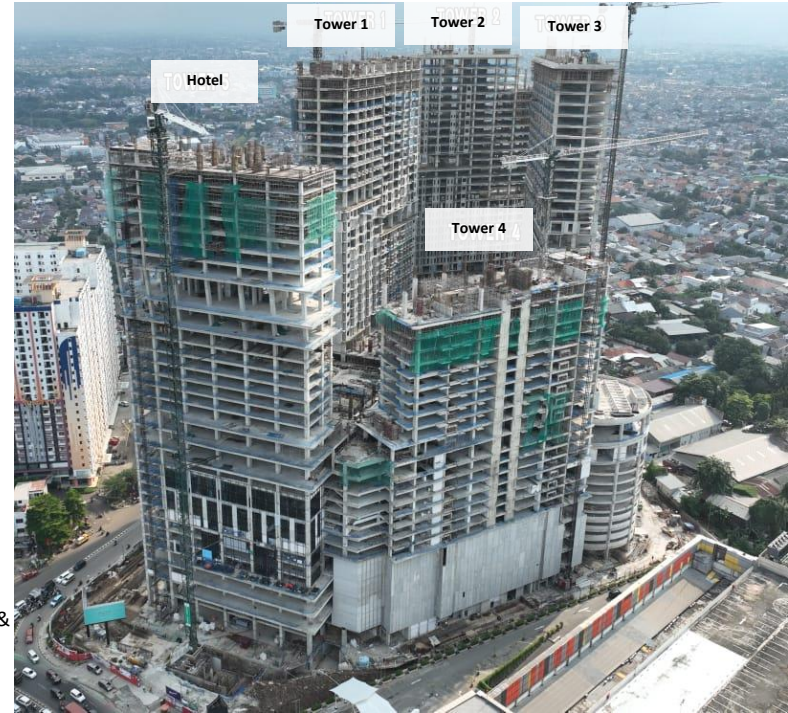
Construction progress as of December 31, 2023
