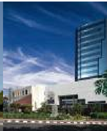
Mandiri Office Tower
